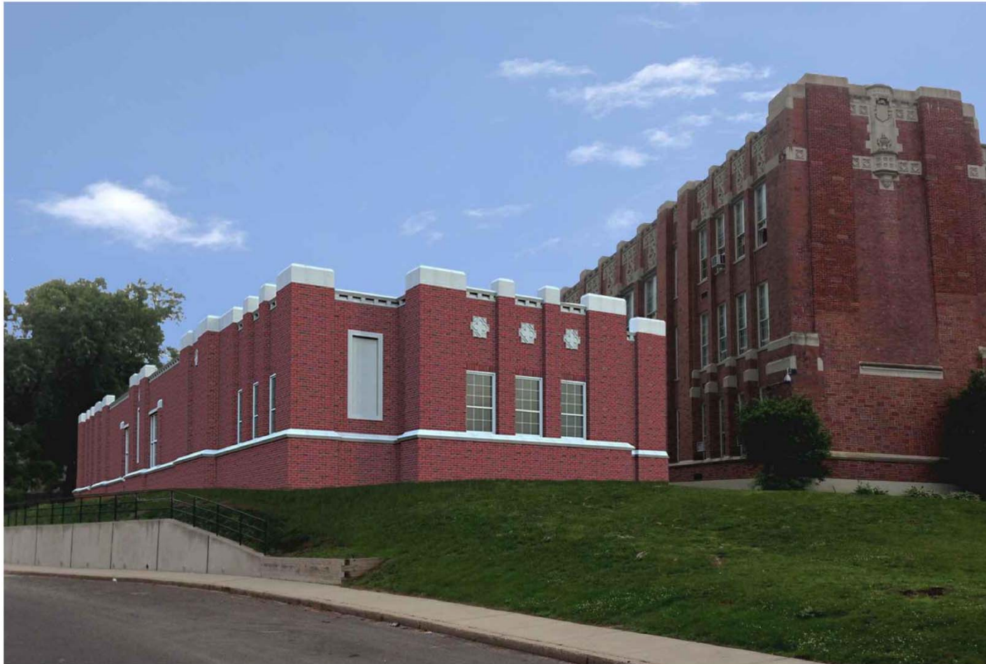
PROPOSED MUSIC & ART ADDITIONS AND ALTERATIONS - NORTHEAST VIEW OYSTER BAY HIGH SCHOOL OYSTER BAY-EAST NORWICH UNION FREE SCHOOL DISTRICT
