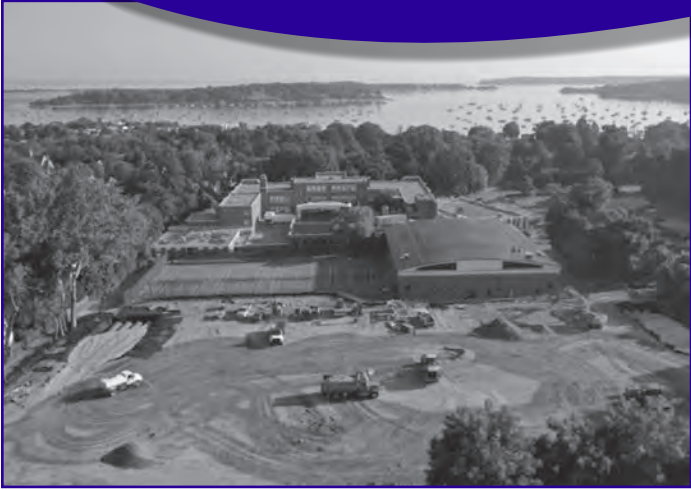
Construction began this summer on the high school's new turf field.
