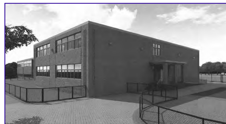
Theodore Roosevelt Elementary School will have a second addition to the building to increase instructional spaces.
