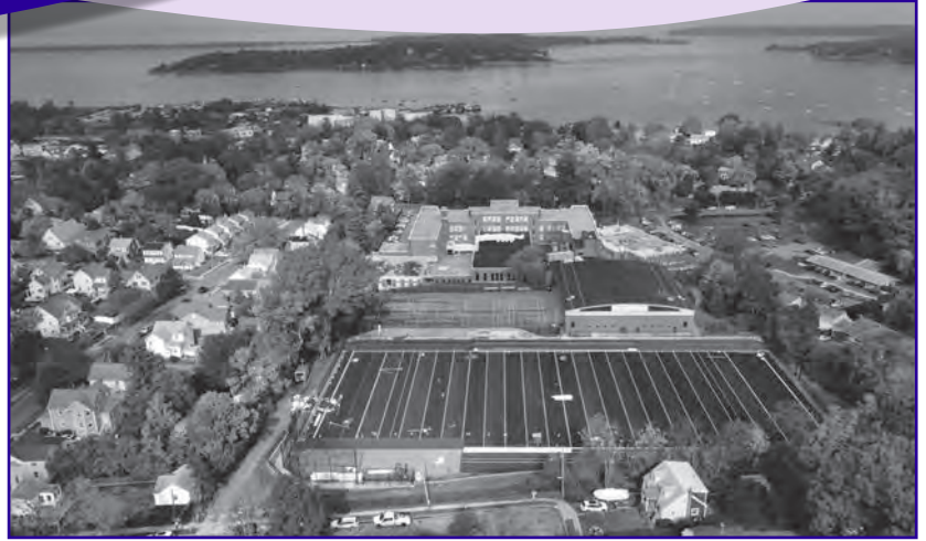
The nearly completed turf field at Oyster Bay High School.
